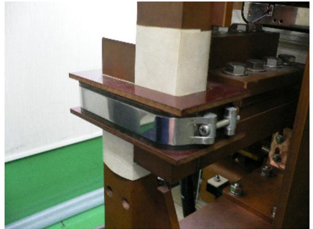
Fig. 3. Photograph of current balancer at output DC bus.
